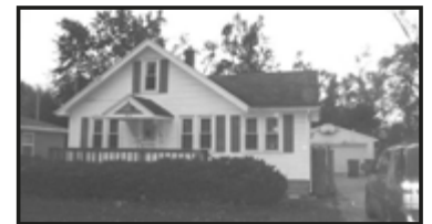
5818 Valencia Blvd, Lansing ***
