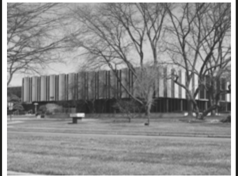
Michigan Education Association Headquarters 1216 Kendale Blvd., East Lansing
