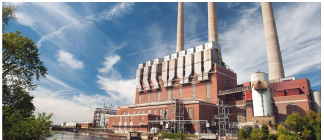
**Eckert Power Station** is the BWL's oldest operating power plant. The 375-megawatt plant's coal-fired generation units were installed over several years, beginning in the mid-1950s. It includes six electric generating units, all of which are scheduled to close by 2020.
