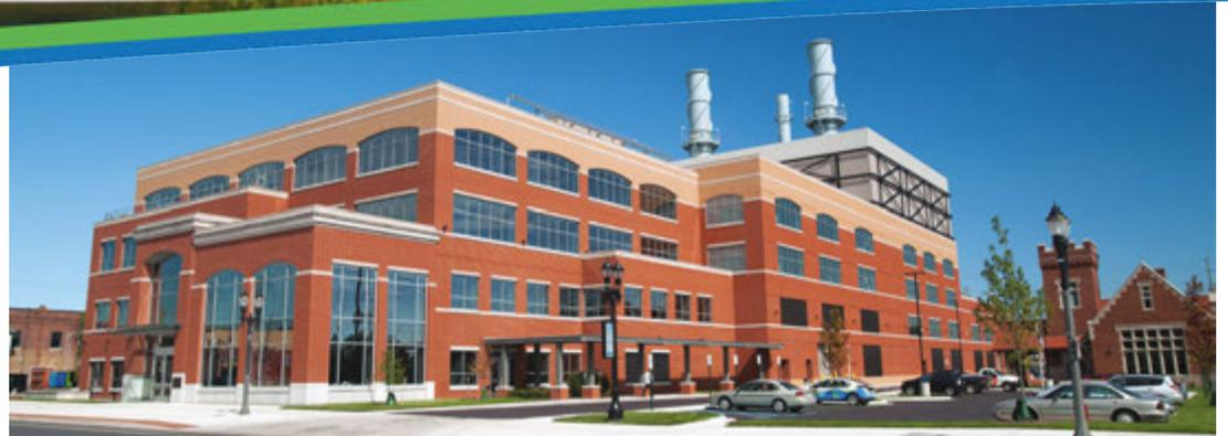
**REO Cogeneration Plant** is BWL's first natural gas-fired power plant – and first new plant in 40 years. The REO Town plant generates up to 300,000 pounds of steam per hour and 100 megawatts of electricity. The plant, winner of many industry awards, is among the most clean and efficient in the U.S.
