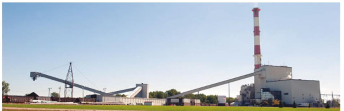
**Erickson Power Station** is located in Delta Township, was completed in 1973 and contains a single coal-fired generator capable of producing 160 megawatts of electricity. It was recently rated one of the most efficient plants of its size in the United States.
