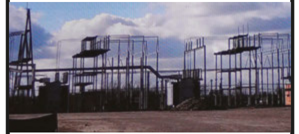
Property: Proposed Substation — Malcolm X and South Washington, Lansing
