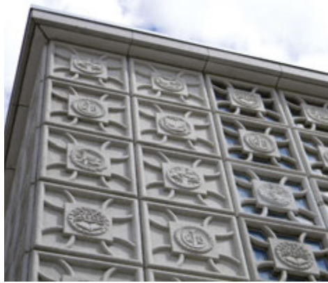
Photo Courtesy of Michigan State Historic Preservation Office
