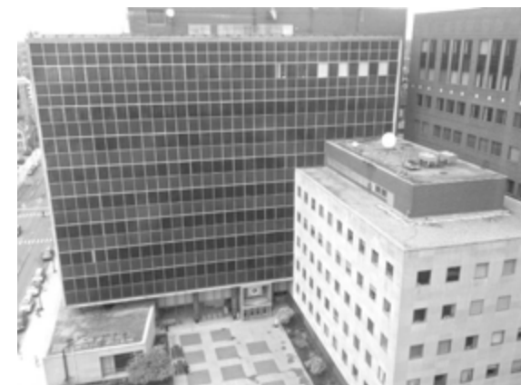
Photo Courtesy of Michigan State Historic Preservation Office
