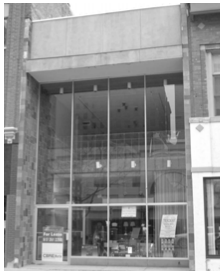
Photo Courtesy of Michigan State Historic Preservation Office
