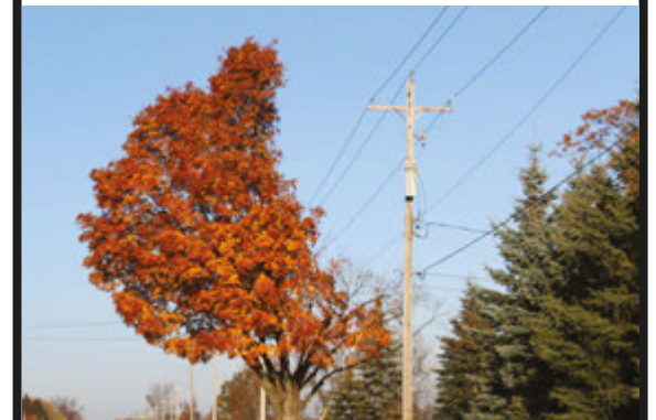
Power lines and trees Everywhere
