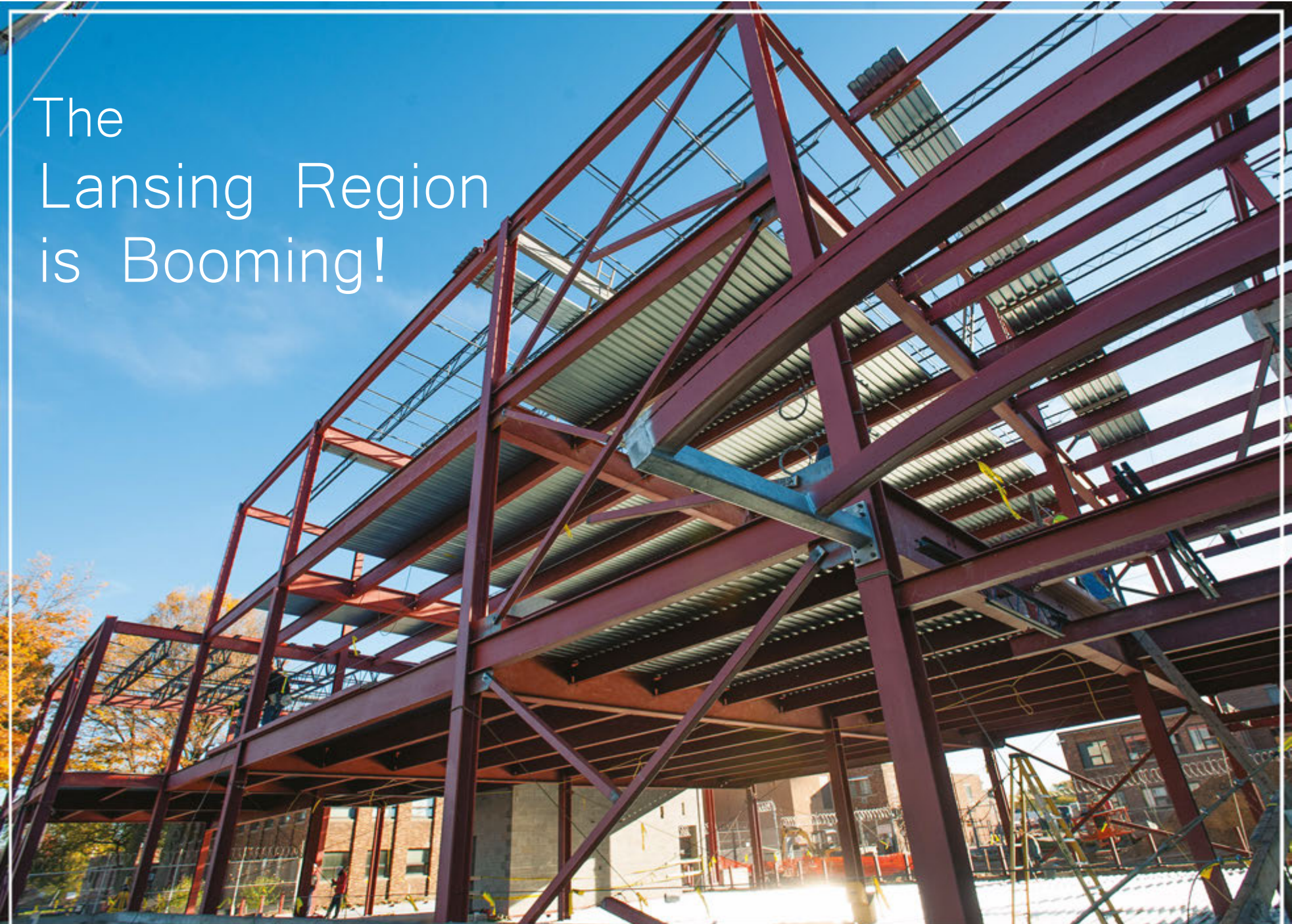
Construction on Emergent BioSolutions' $108M campus expansion
