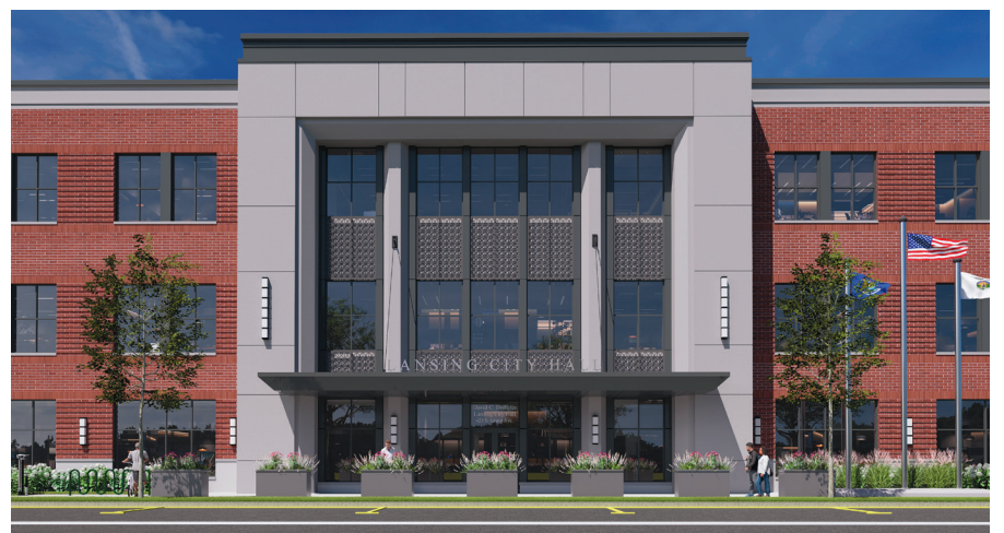
Another look at Lansing's new City Hall.
