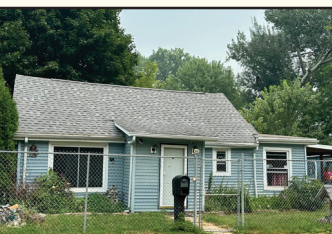
Property 3352 - Lansing 229 Dunlap St.
